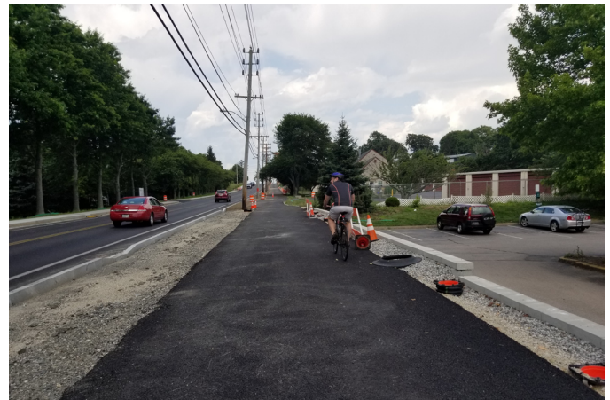
Photo of the Newport Connector Trail along JT Connell under construction
