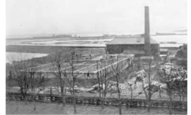
1910 Newport RI Water Treatment Plant
