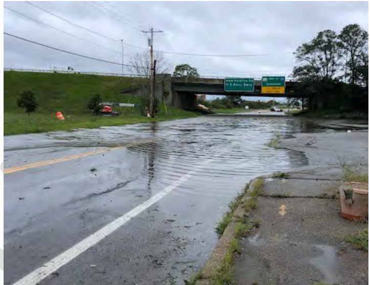
Flooding at JT Connell Highway on Sept 2, 2021 after the remnants of Hurricane Ida.
