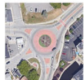
West Warwick Roundabout
