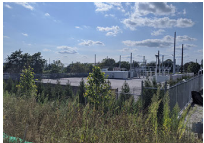
Natural systems can be integrated into the Maker subdistrict to improve resiliency and buffer noxious uses from more publicly-oriented commercial uses.
