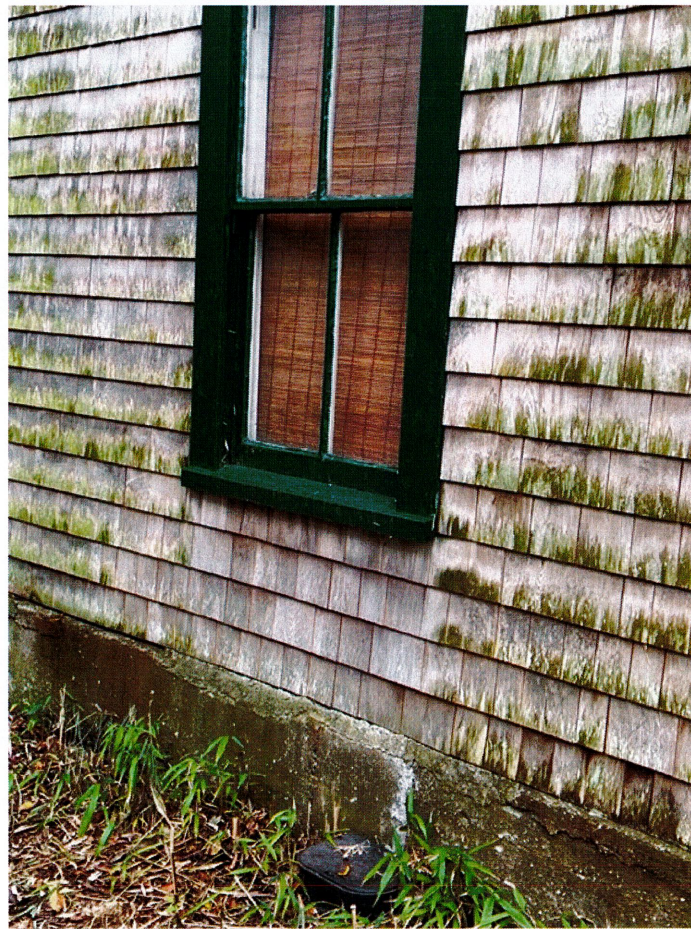
Figure 4 - Detail at window
