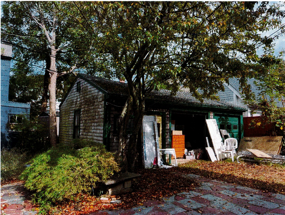
Figure 2 - Exterior of Garage
