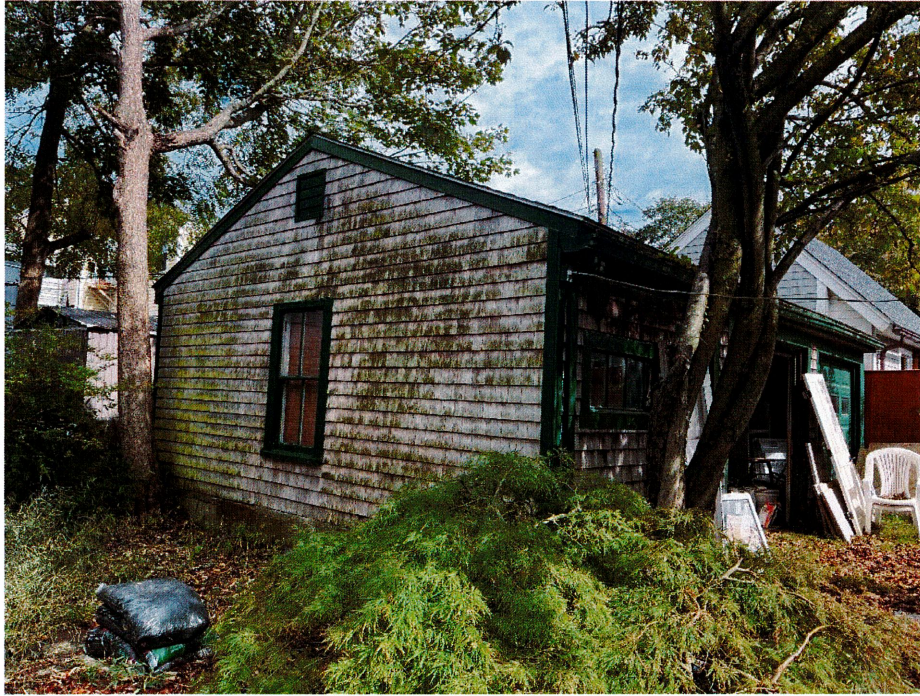
Figure 3 - Exterior of Garage
