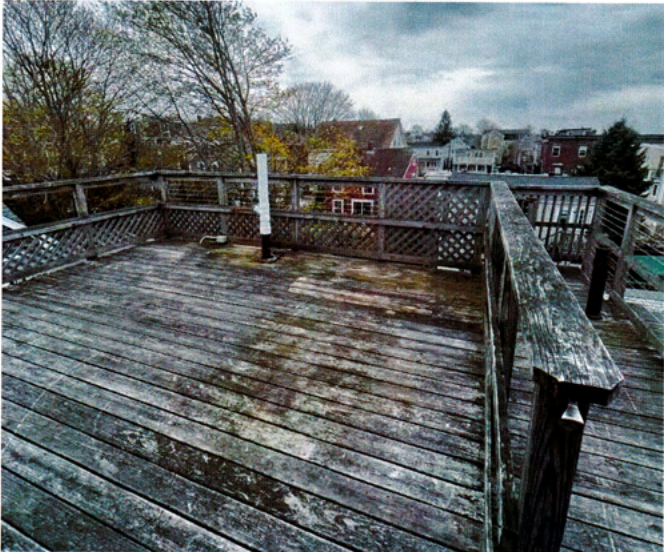
03: EXISTING VIEW - ROOF DECK
