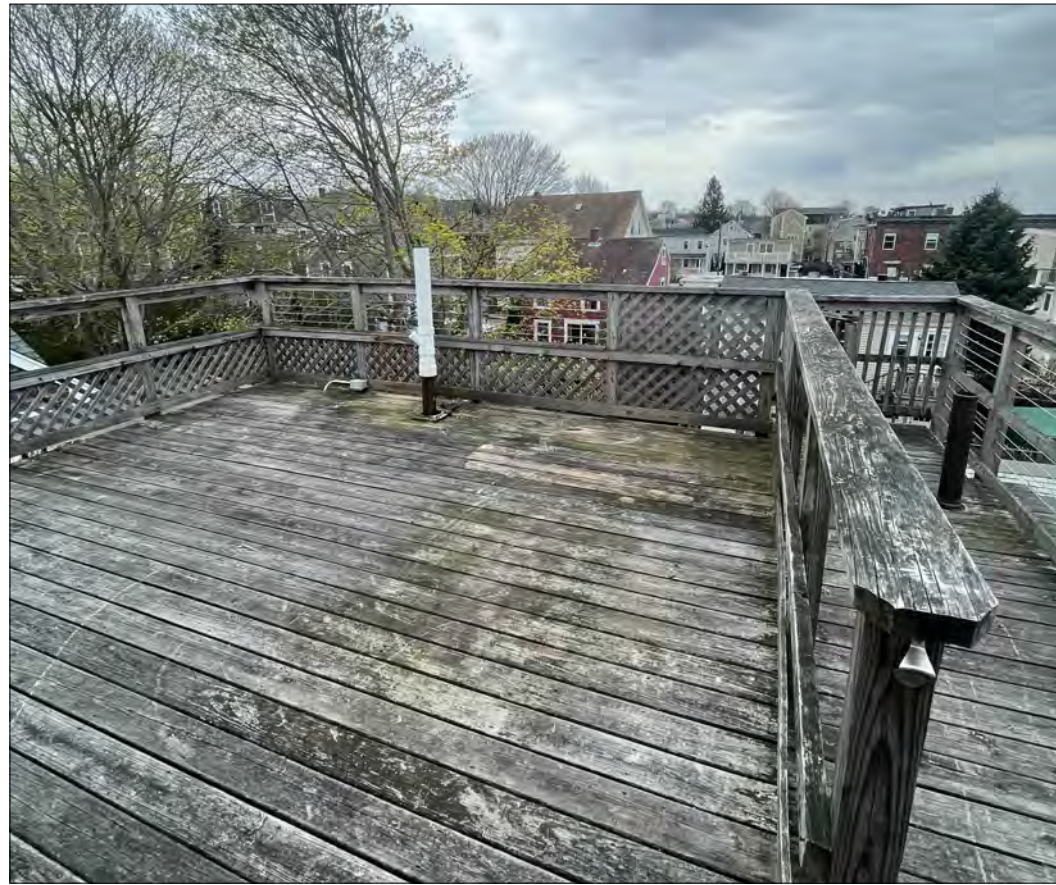
O3: EXISTING VIEW - ROOF DECK
