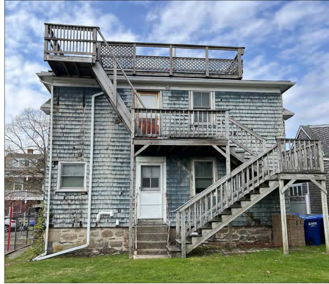
O2: EXISTING VIEW - REAR
