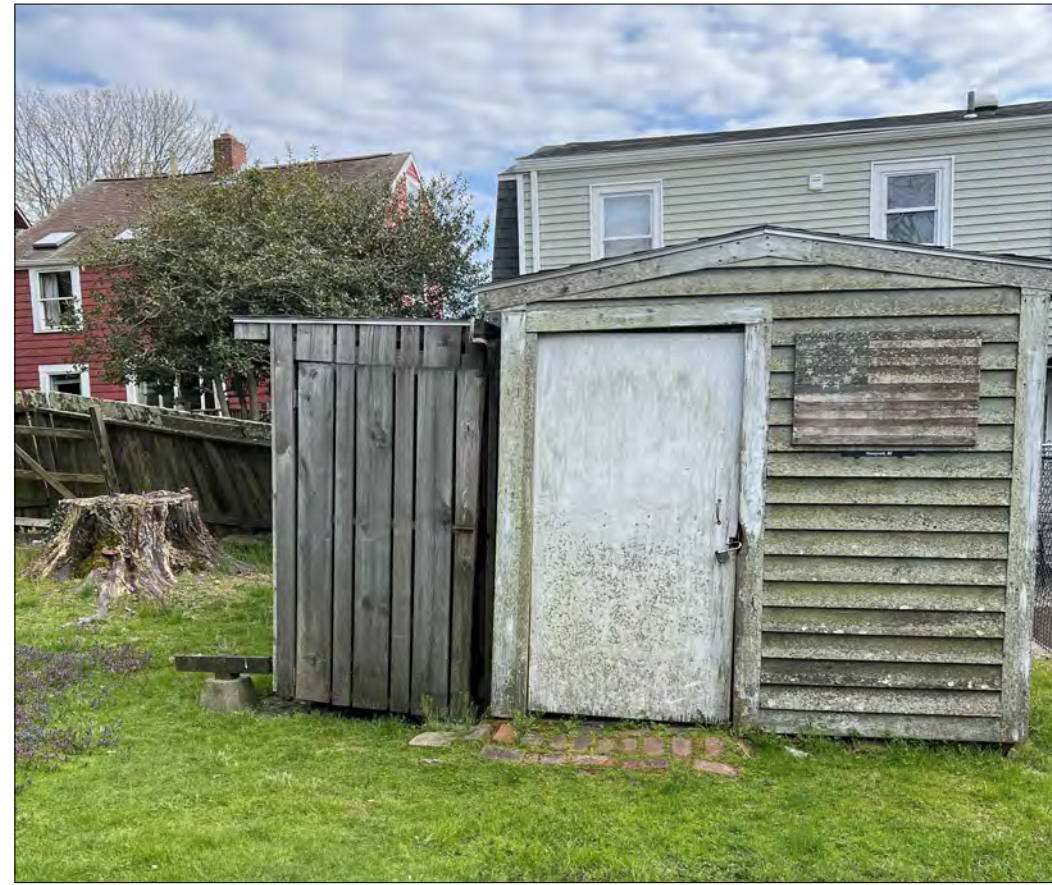
O4: EXISTING VIEW - SHED
