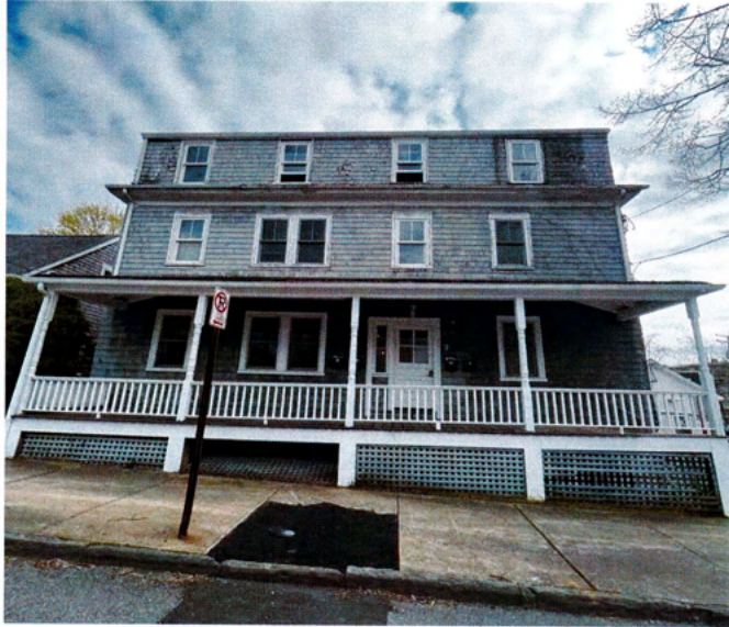
01: EXISTING VIEW - FRONT
