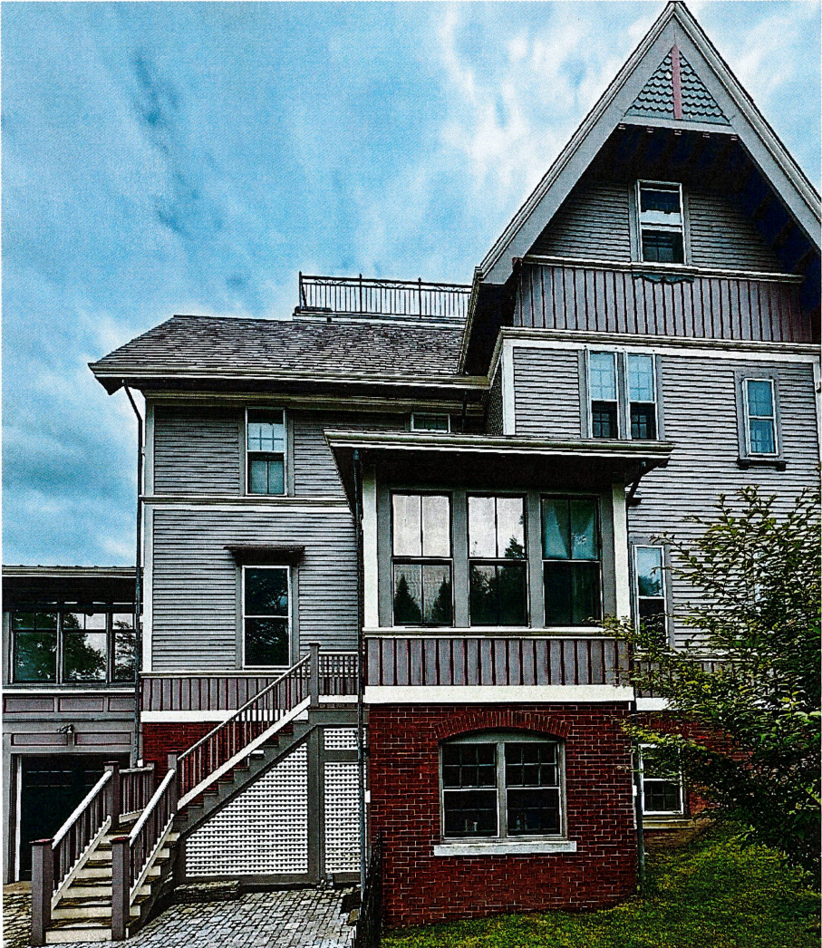
6. NORTH FAÇADE (REAR) CATHERINE STREET
