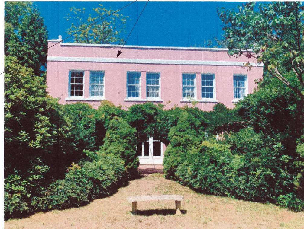
MAJOR CRACKS IN STUCCO
