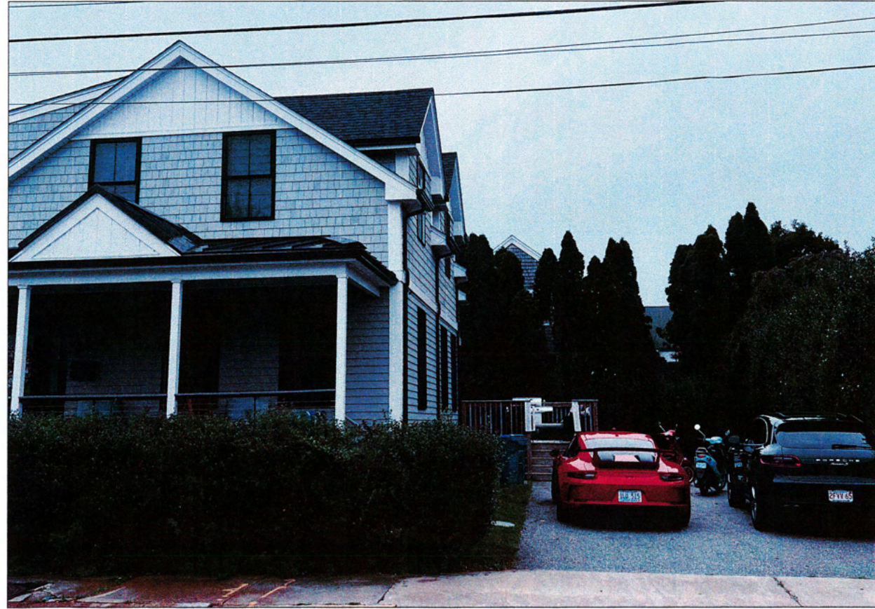
O4: EXISTING DECK & PARKING
