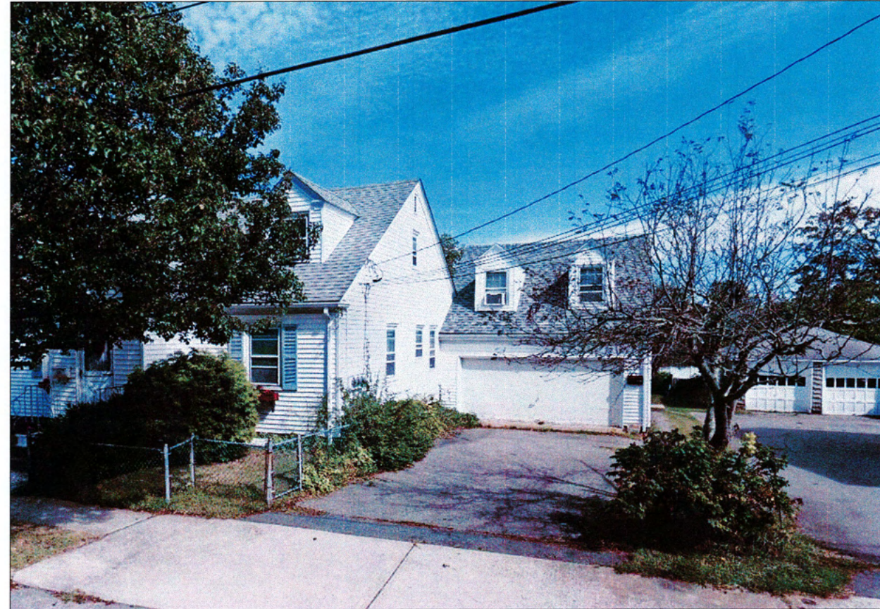
O4: EXAMPLE ON ROSENEATH AVENUE, NEWPORT
