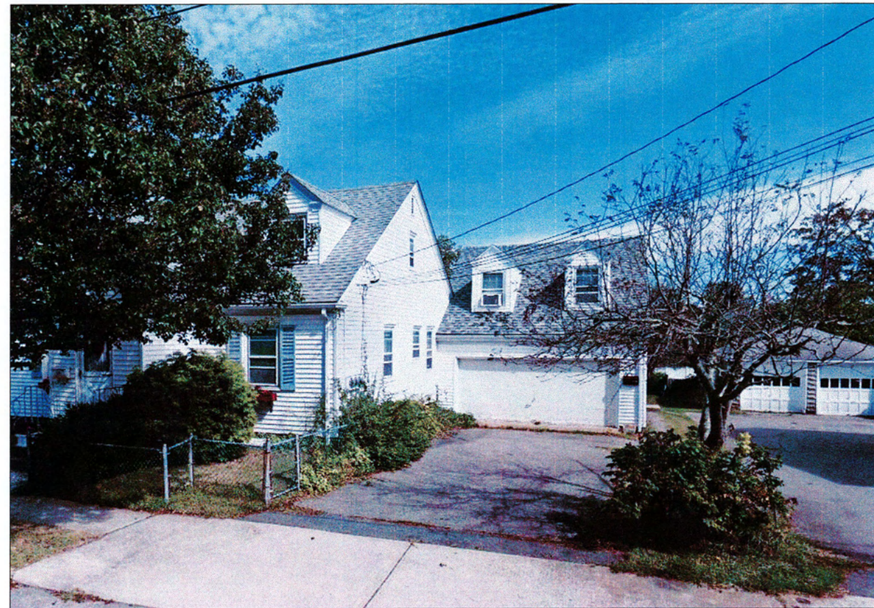
O4: EXAMPLE ON ROSENEATH AVENUE, NEWPORT
