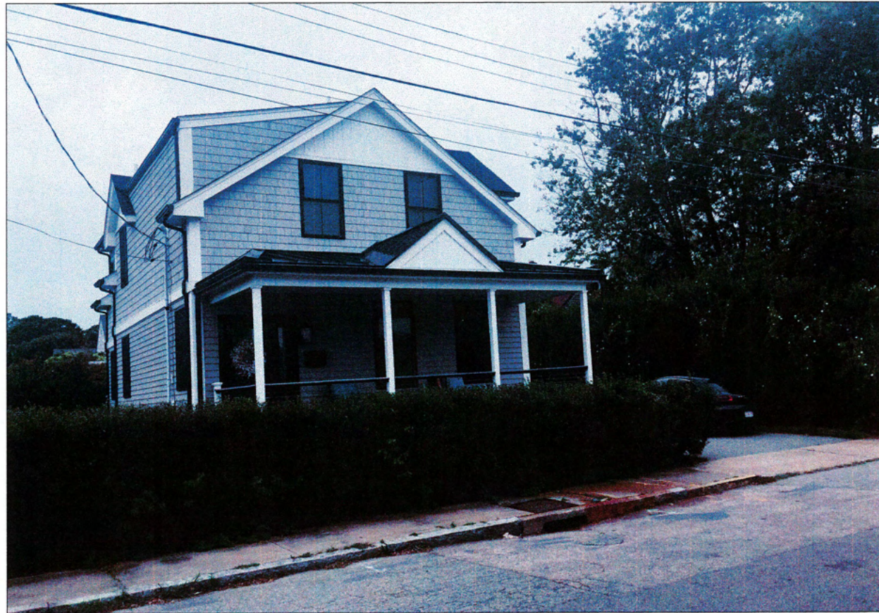
O3: EXISTING FRONT PORCH & VEGETATION
