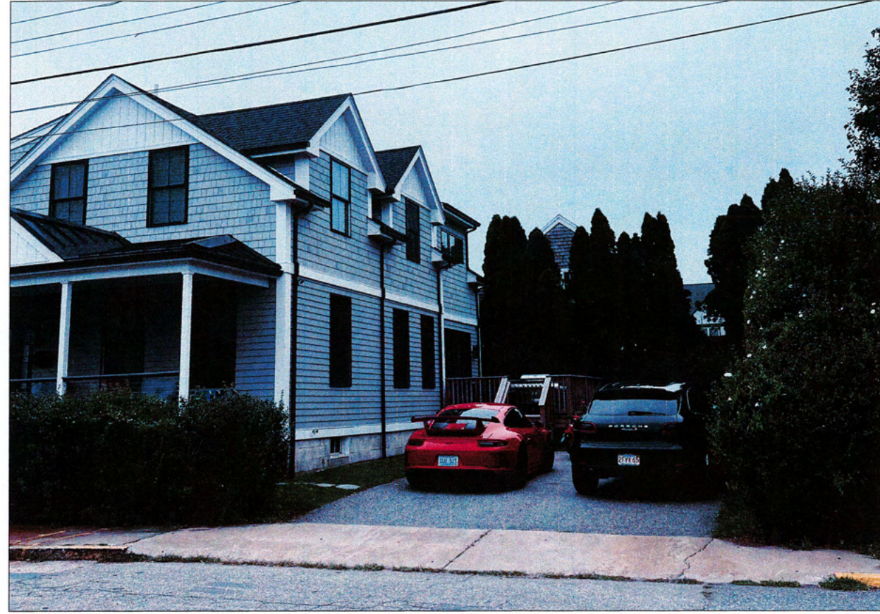
O2: EXISTING STREETVIEW - RIGHT
