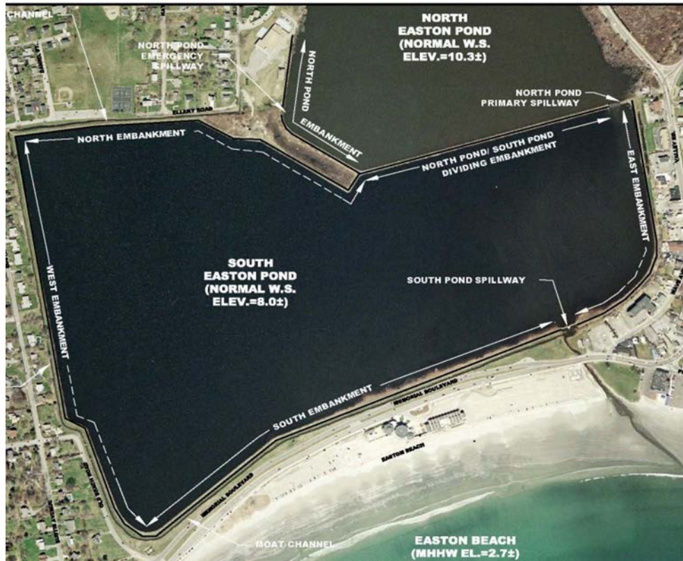
Figure 2: Aerial view of the Easton Pond Dams.
