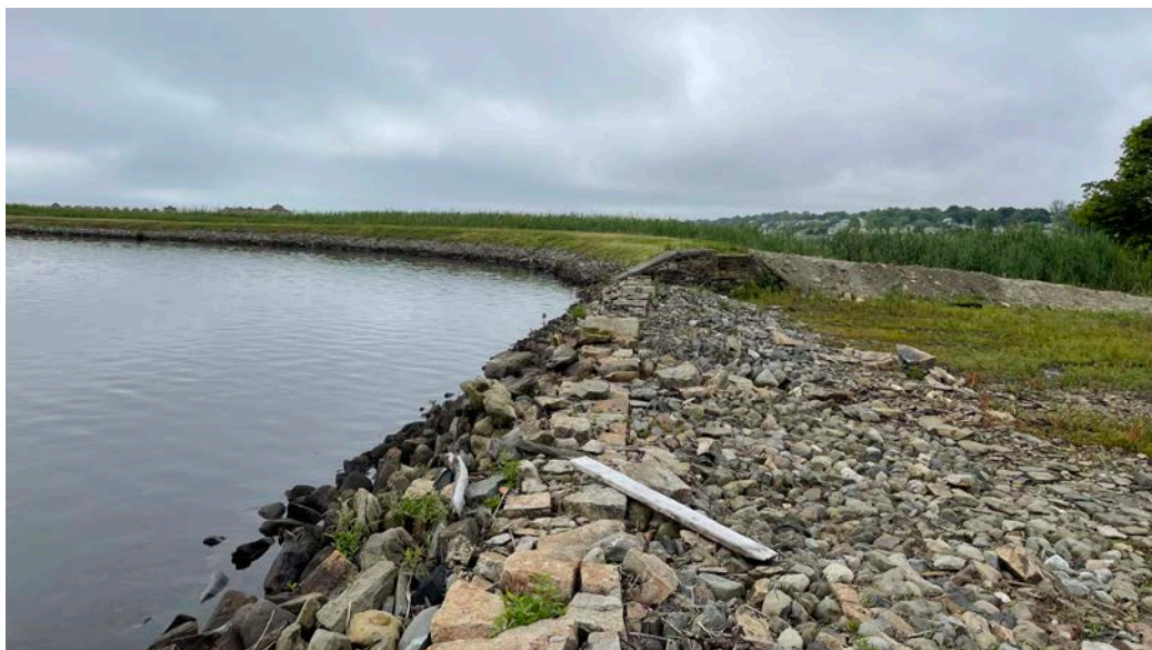
Figure 10: North Easton Pond Auxiliary Spillway
