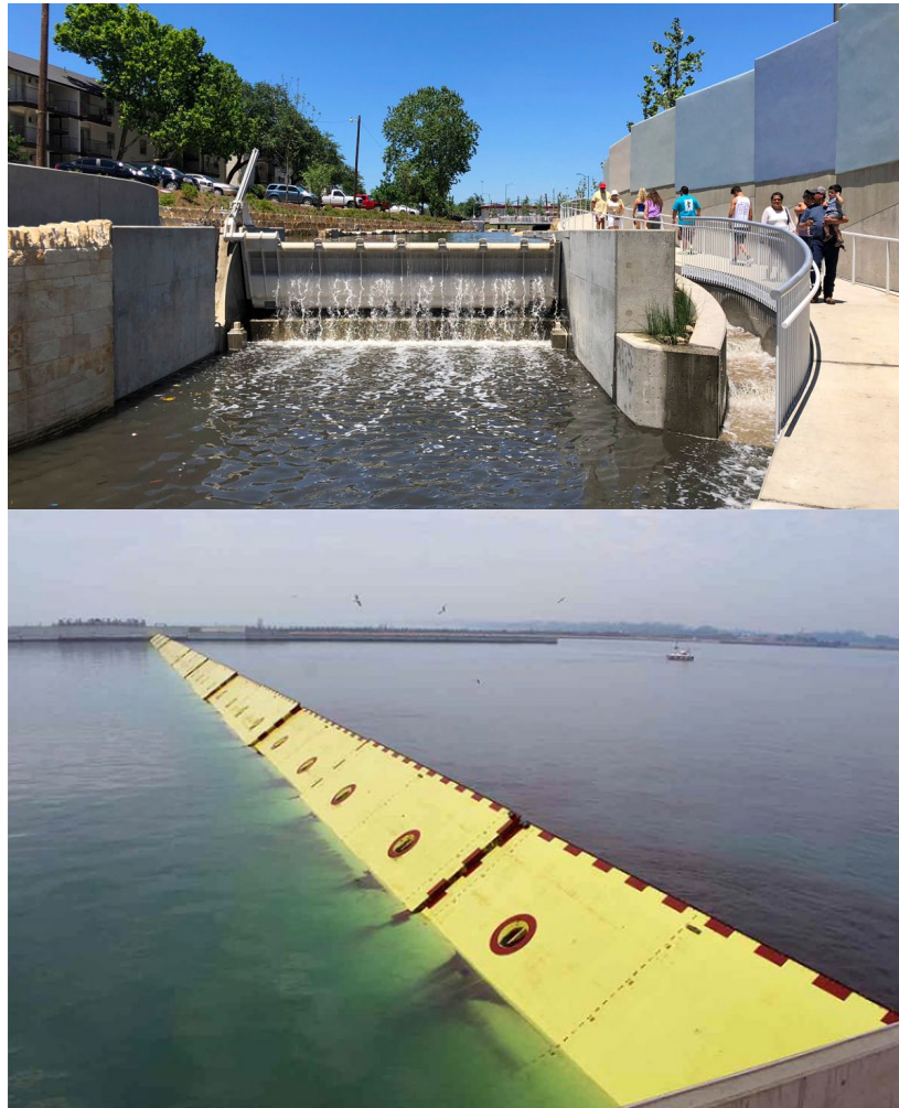
Figure 6: Crest Gate Examples (top http://steelfabinc.com/product/crest-gates/ ) (bottom: https://www.designboom.com/architecture/mose-flood-barrier-venice-storm-alex-10-05-2020/ )
