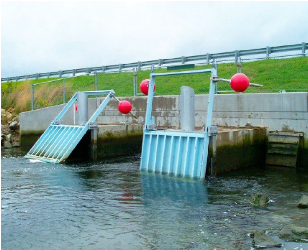
Figure 7: Tidal gate example ( https://watermanusa.com/products/large-custom-gates/self-regulating-tide-gates/ )
