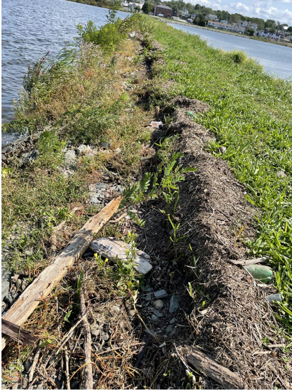
Figures 1 and 2: Embankment damage following Hurricane Ida on the NEP embankment (Photo provided by City)
